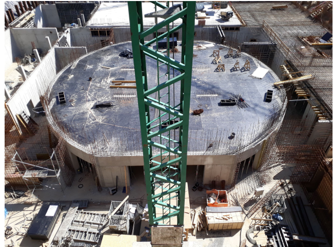
Figure 1: Warsaw State Music School Complex Nr 1 Construction Site (2018.05.08) ©Konior Studio
