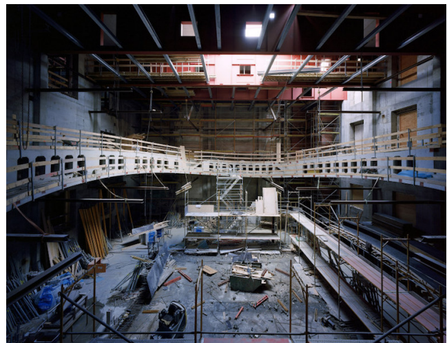
Figure 3: Pierre-Boulez-Saal Under Construction
