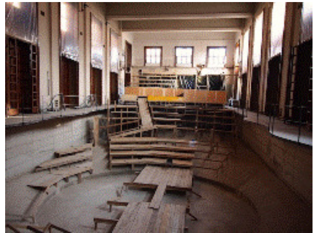
Figure 3: Chamber Hall Under Construction
