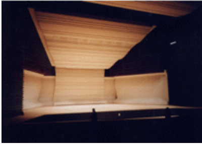
Left: The stage sound reflection panel system set up on stage
