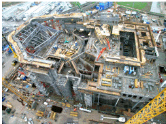
Figure 1: Danish Radio Construction Site
