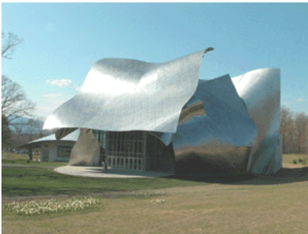
Fisher Center at Bard College Exterior
